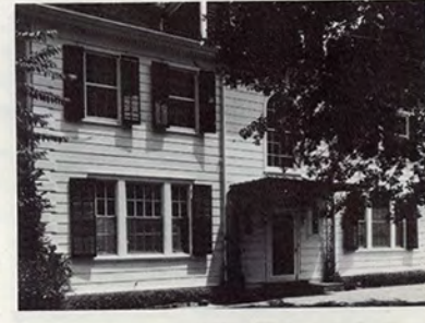
8 Will L. Clayton Summer House 3376 Inwood Drive - Country Club Estates 1924/Briscoe & Dixon, arch.
