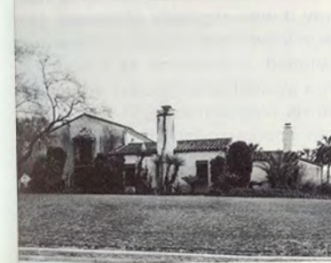
2 Mrs. Harmon Whittington House 2416 Pine Valley Drive 1935/John F. Staub, arch.
