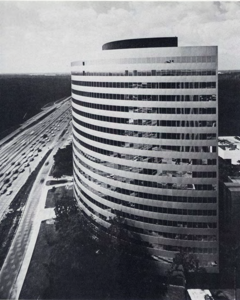
LEFT: U.S. Home Building on West Loop South in Houston, designed by the Houston firm Caudill Rowlett Scott. BELOW: Century Center on Loop 410 in San Antonio, designed by the Houston firm 3D/International.
